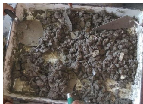
Fig. 2: Mixing of cement, sand, aggregate & ceramic with water.
